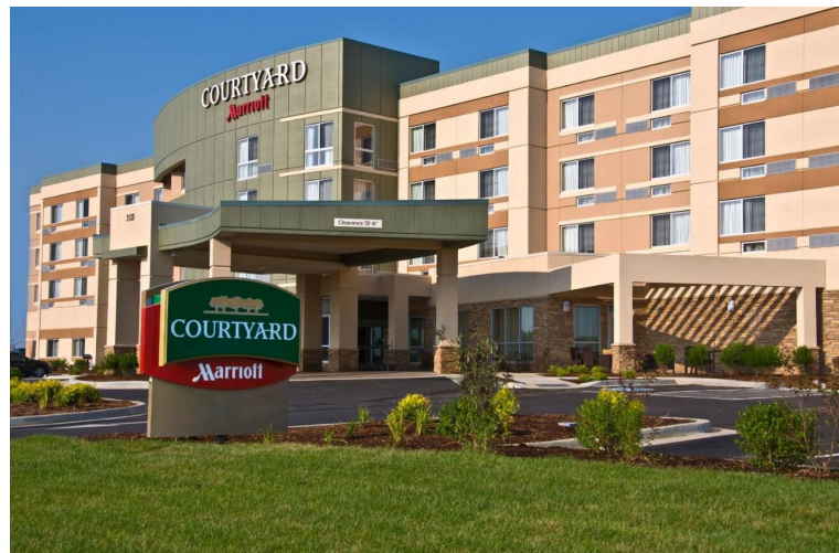
Courtyard by Marriott Owensboro 3129 Highland Pointe Drive 270-685-4140
